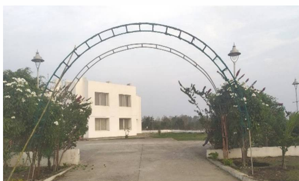
Arch fabricated by using scrap materials for Horticulture Deptt.
