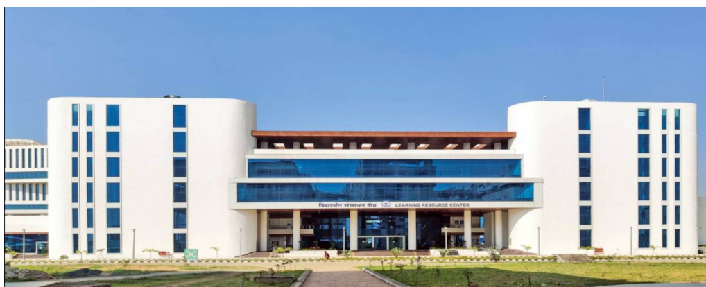
Figure 1. The Learning Resource Center (LRC) Building
